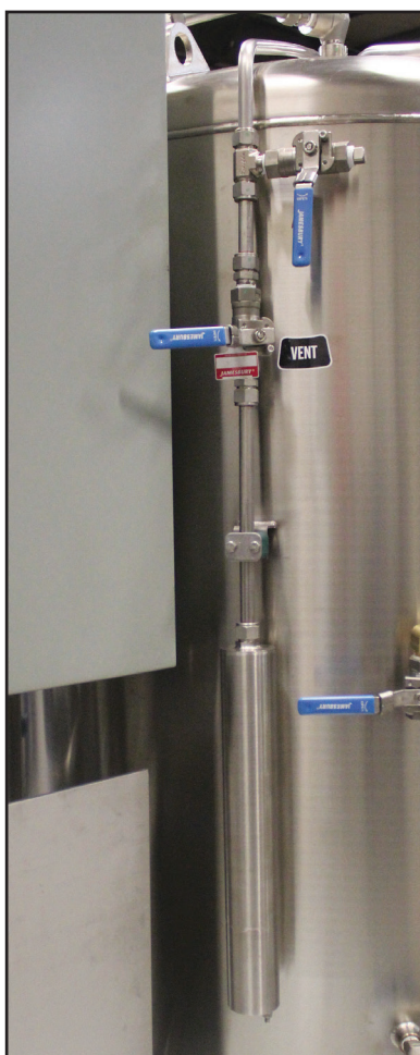
Figure 21 - Muffer on vent/full trycock plumbing circuit
