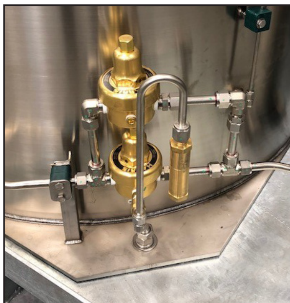
Figure 16 - Dual PB regulators
