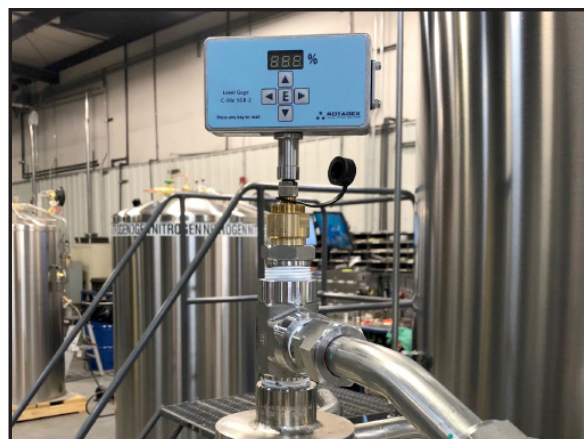
Figure 22 - C-Stic Liquid Level Gauge
