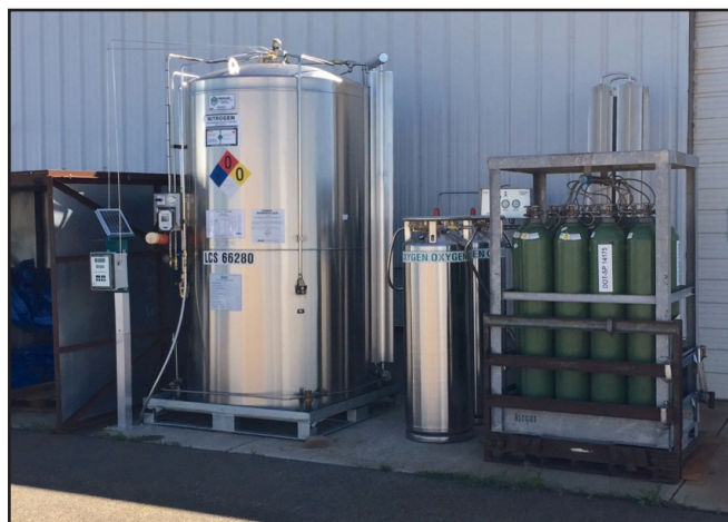
Figure 25 - Perma-Max 3300HP with external pressure build vaporizer
