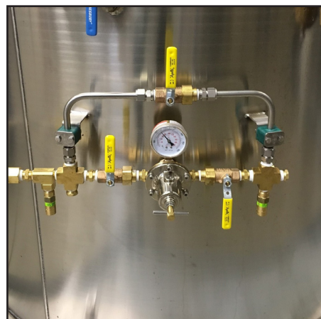
Figure 9A - Regulating manifold
