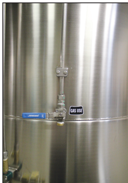
Figure 9 - Gas Use ball valve
