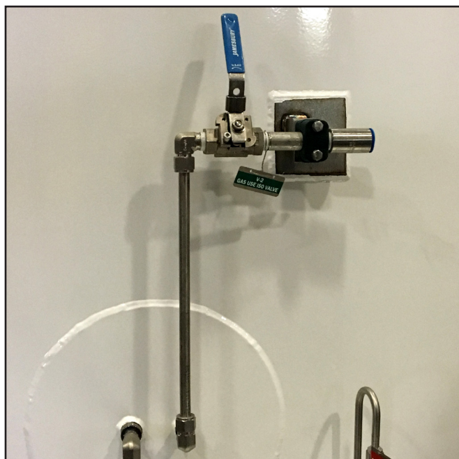
Figure 32 - Gas Use Valve (V-2)
