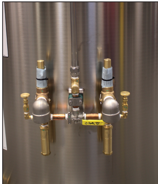
Figure 20 - Diverter valve, Bleed-off valve, Primary Relief valve (top) and Secondary Relief valve (bottom)
