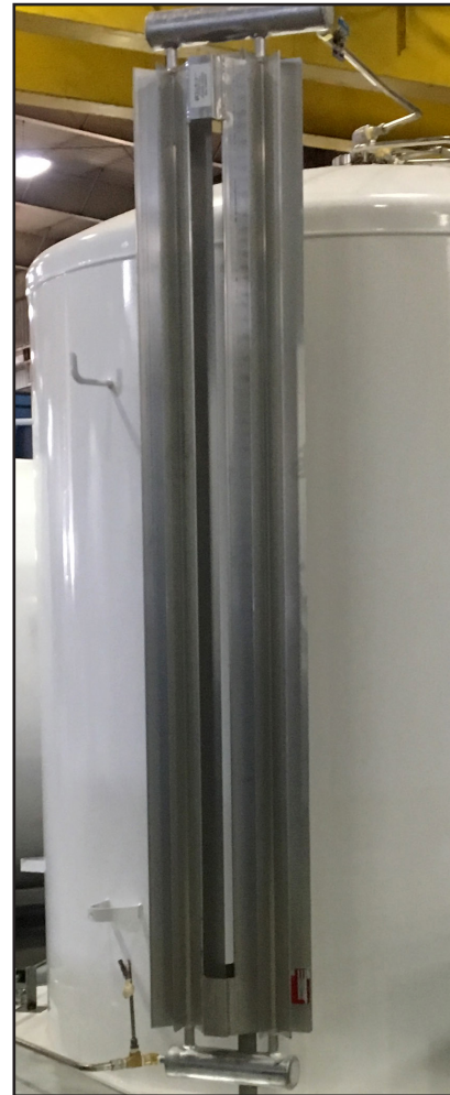
Figure 28 - Pressure Build (PB) Vaporizer
