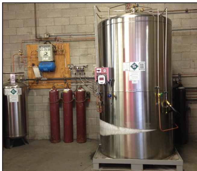
Figure 27 - Indoor Installation of a Perma-Max 3300HP tank
